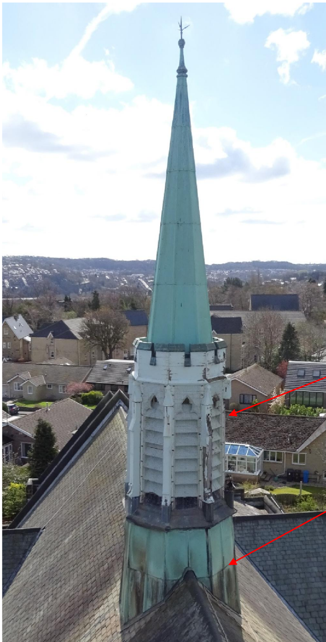
St Andrews Psalter Lane Church Spire in April 2022 – Deteriorated condition of timber and buttress part that has fallen off. Insecure copper cladding
