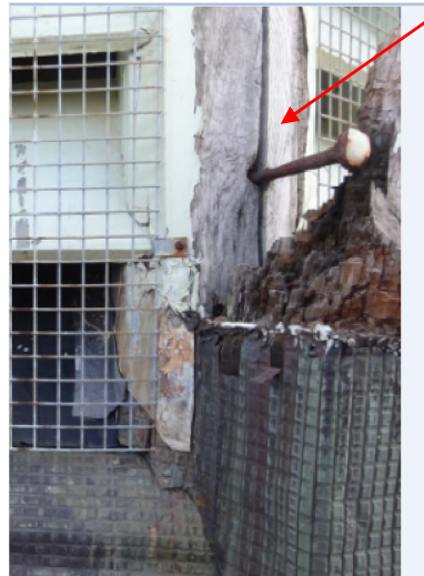
St Andrews Psalter Lane Church Spire in April 2022 – Note that parts of corner buttress pieces are rotten and parts are missing.
