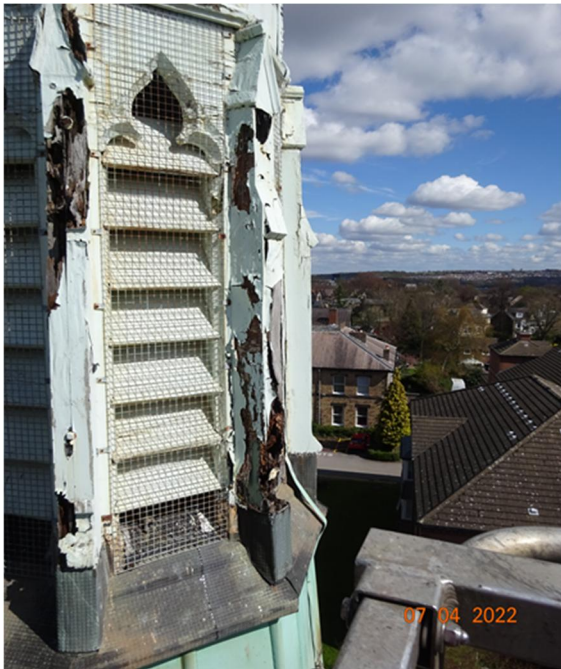
St Andrews Psalter Lane Church Spire in April 2022 – Note that parts of corner buttress pieces are rotten and parts are missing.
