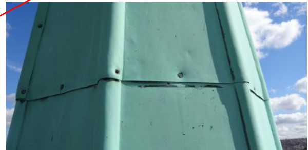
St Andrews Psalter Lane Church Spire in April 2022 – Deteriorated condition of timber and buttress part that has fallen off. Insecure copper cladding
