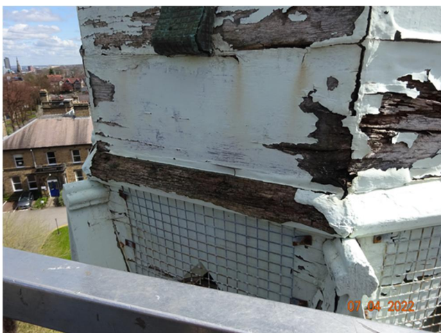
St Andrews Psalter Lane Church Spire in April 2022 Moulding is rotten and has become detached.
