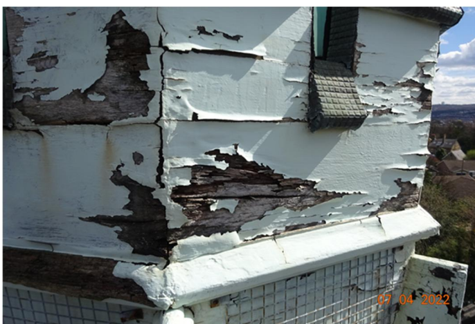
St Andrews Psalter Lane Church Spire in April 2022 – Deteriorated condition of Castellated crown. Artificial lead has been used to repair the castellation valley
